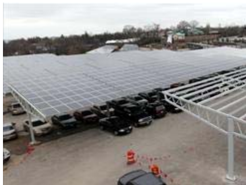
Ernest Coleman, The Cincinnati EnquirerSolar panels installed at the Cincinnati Zoo and Botanical Garden parking lot will generate 20%
